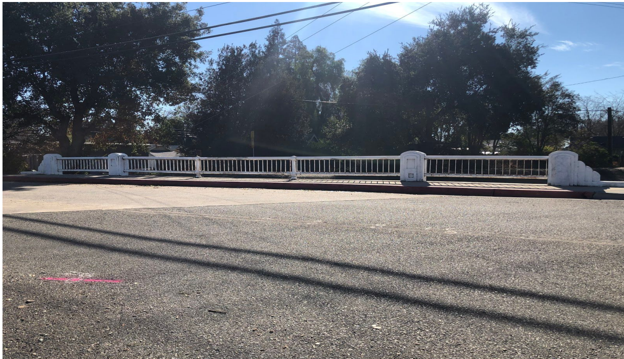
Stoddard Avenue Bridge with Art Deco masonry
