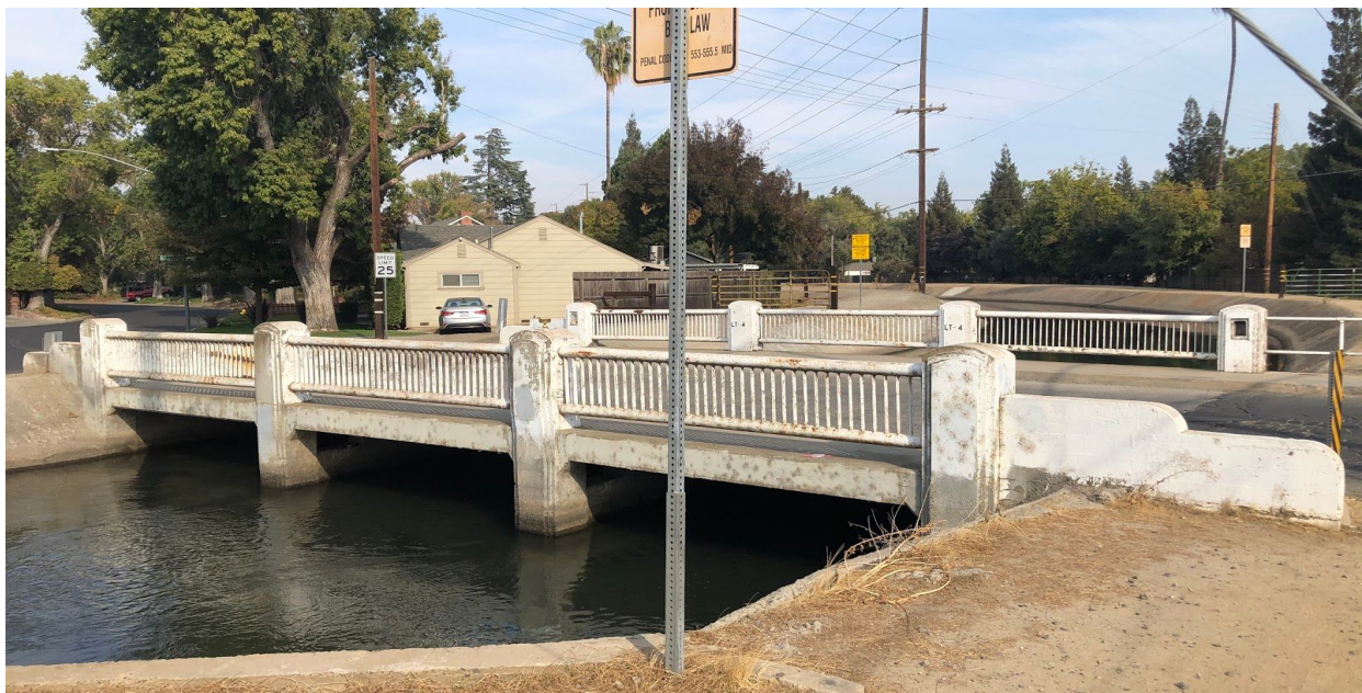
Johnson/Ila Ave Bridge with Art Deco masonry
