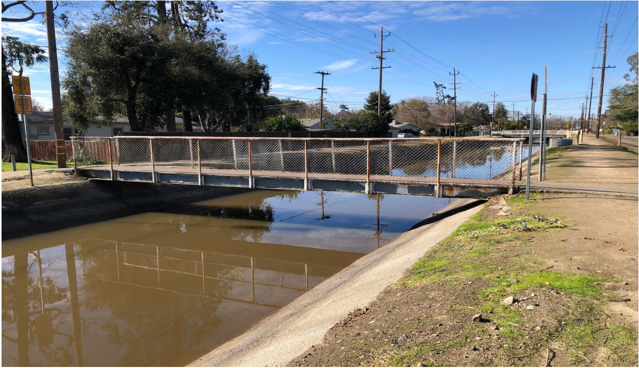
Magnolia Avenue Footbridge #2
