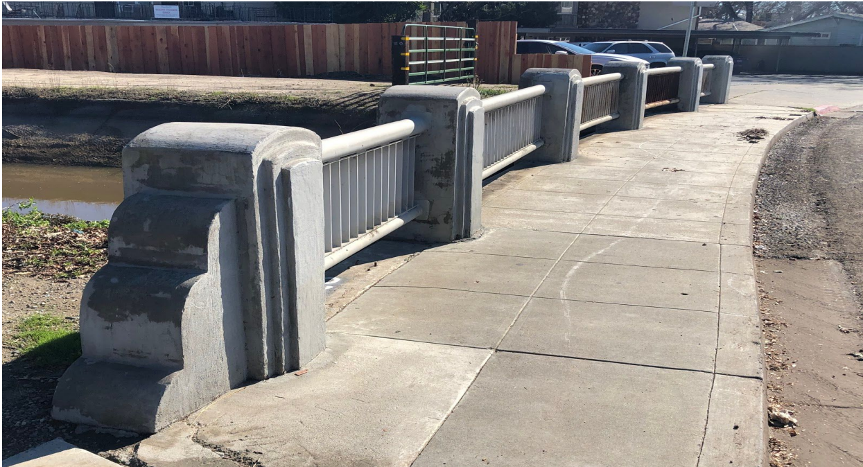
College Avenue Bridge with Art Deco masonry
