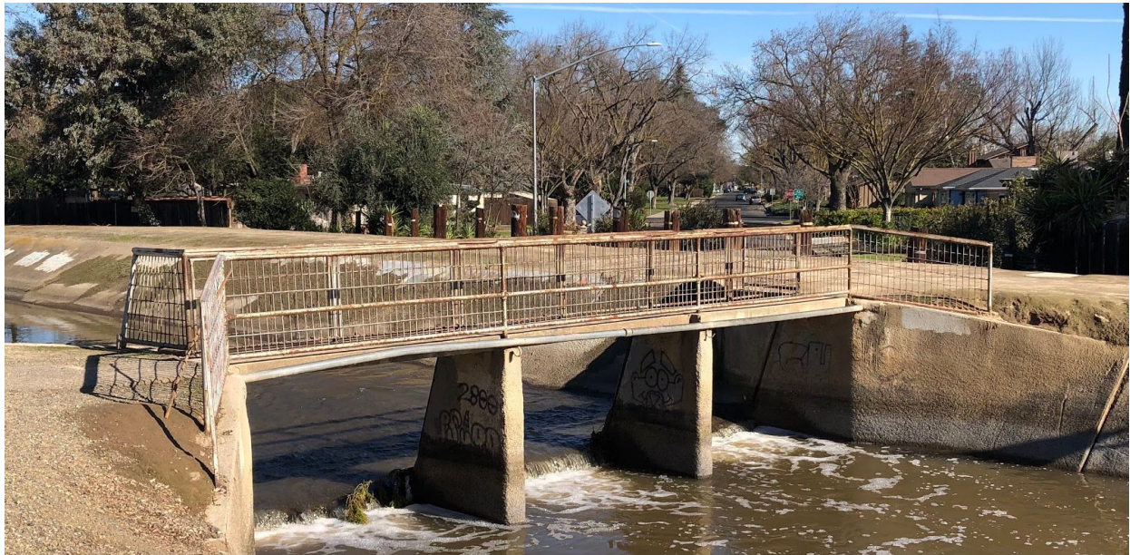
Helen Avenue Footbridge #1
