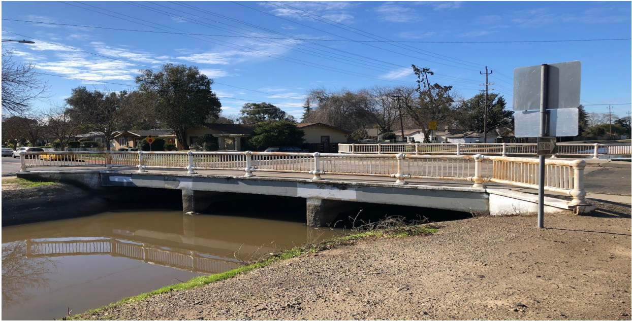
Sycamore Avenue Bridge - no Art Deco masonry
